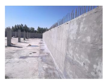
Xypex Concentrate was applied to the interior surface of the treatment tanks spanning 2,289 m². Xypex Concentrate penetrates into the concrete where it chemically reacts, forming an insoluble crystalline structure that seals micro-cracks and capillaries, preventing water ingress. The Xypex crystalline also increases the concrete's chemical resistance by significantly reducing the ingress of deterioration causing substances like chlorides and sulphates.
